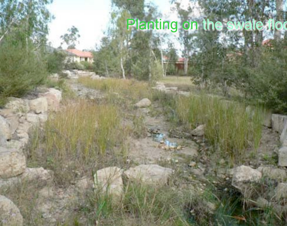
Planting on the swale floor for pollution control
