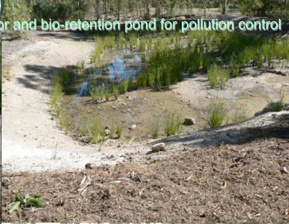
Planting on the swale floor for pollution control
